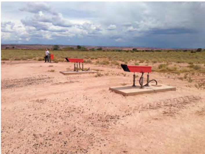
Two box VASI system. Facilities were in fair condition.
