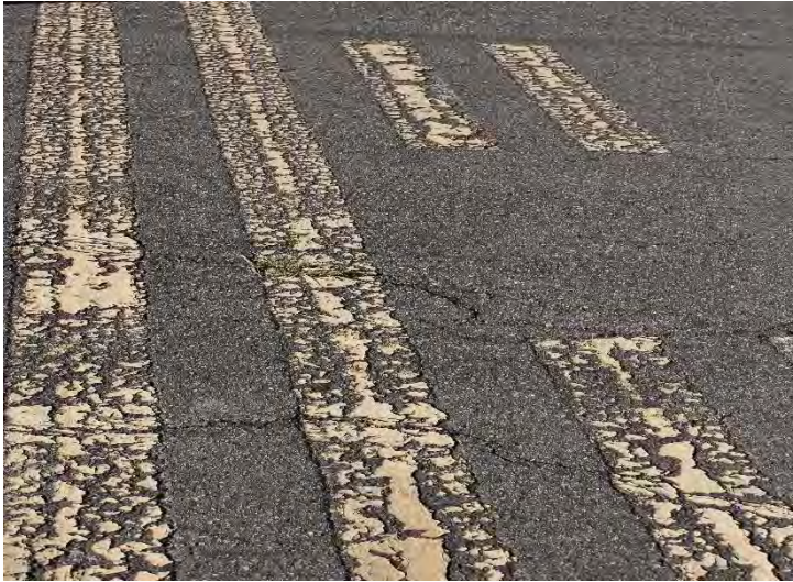
Pavement markings are badly faded.
