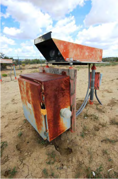
VASI System. Poor condition.
