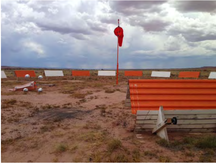
Windsock and segmented circle. Facilities were in good condition.
