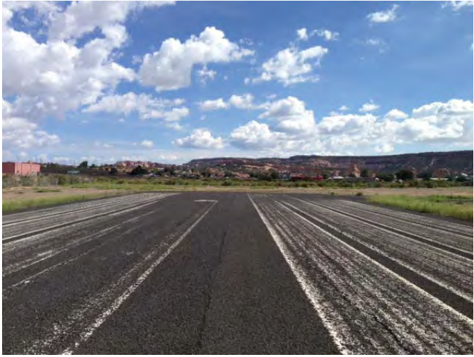
Approach end of Runway 02 looking to the North. Markings are very poor and faded.
