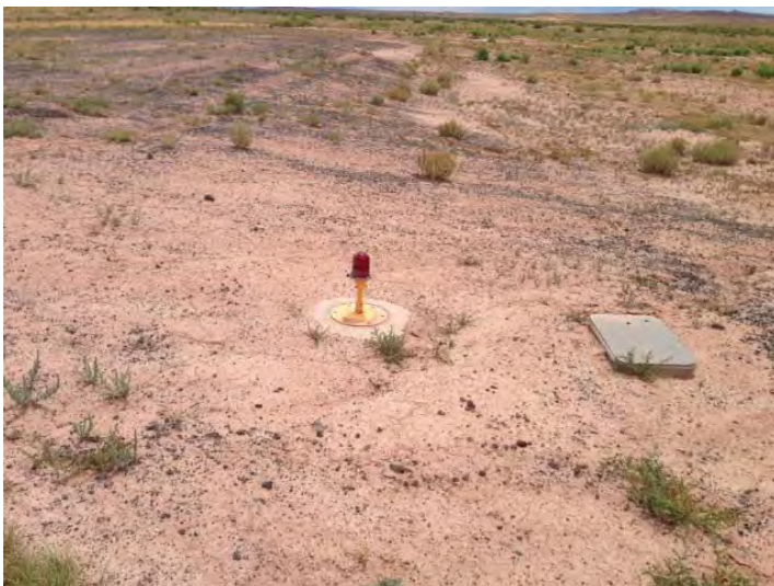
Runway lighting appears to be in fair condition. Lighting system appears to be in cans as opposed to stake mounted.
