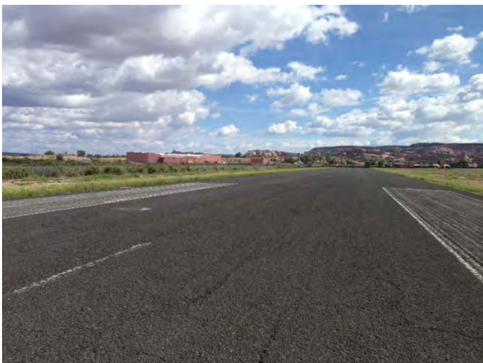
Threshold of Runway 20 looking to the South. Pavement cracking is prevalent throughout the length of the runway.
