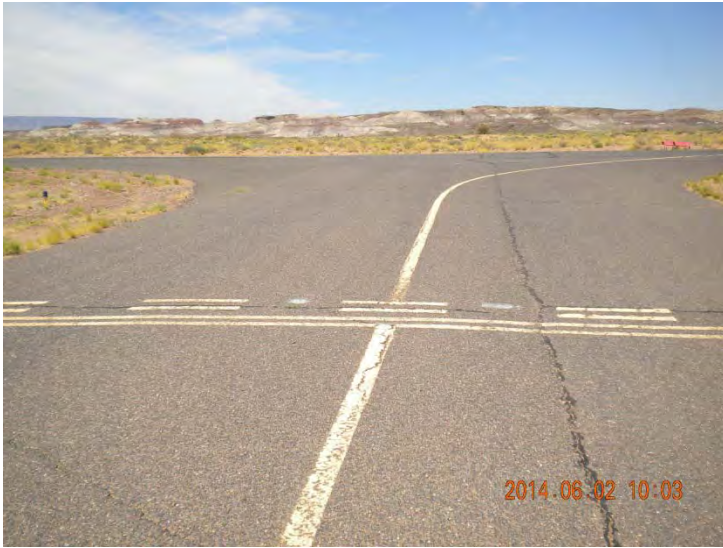
Taxiway Lead-in Line and Hold Bars located on the South end of the runway.
