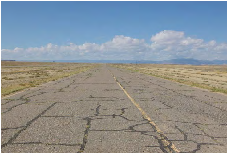
Parallel Taxiway with widespread cracking. Pavements is fair condition, with previous crack seal applications in evidence.
