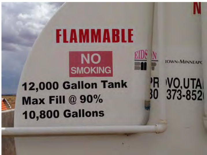
Close up of 12,000 Gallon Jet-A fuel tank.
