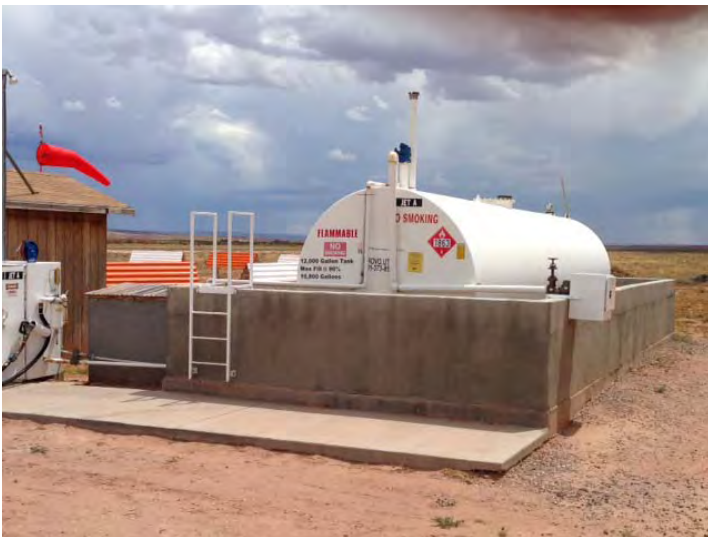
Fuel farm and containment structure. Privately owned by Air Med operator.
