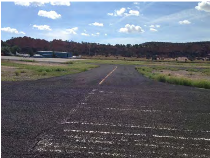
Taxiway tie in to Runway 20. Pavement in fair condition. Markings are very poor and faded.
