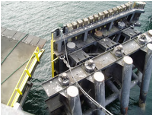
Wing Wall Ground Anchors Figure 26
