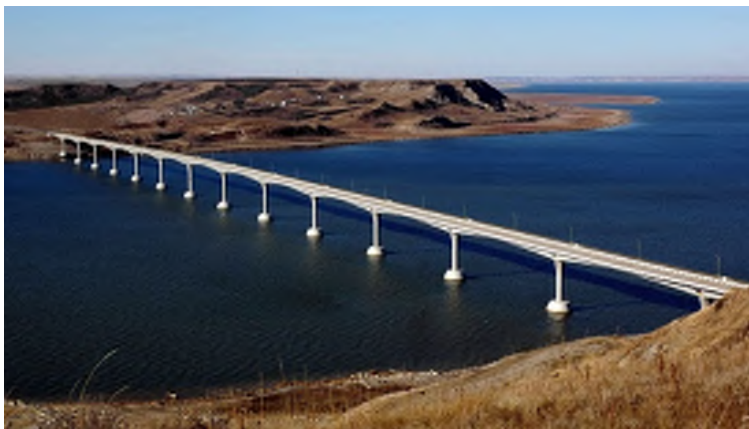
Figure 7. Four Bears Bridge (above)
