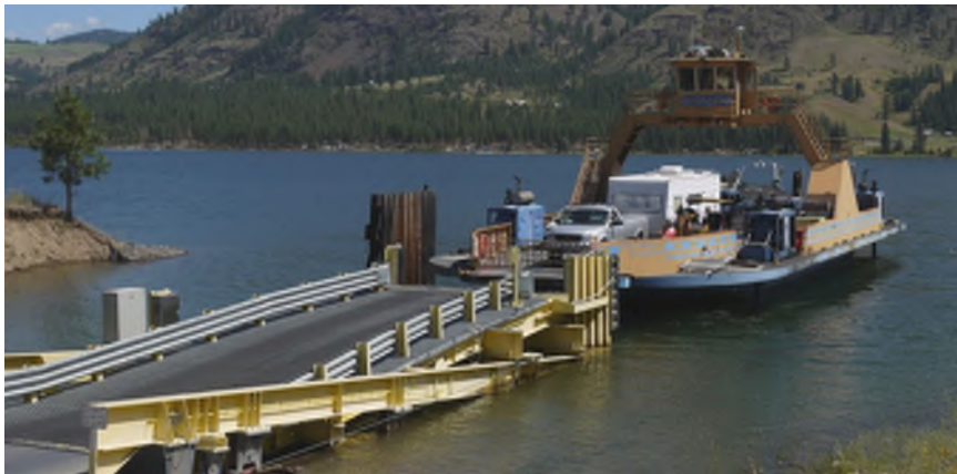
Movable Rail Dock
