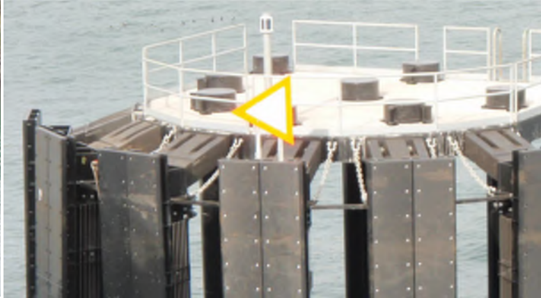
Figure 25 Fixed Dolphin with Navigational Aids
